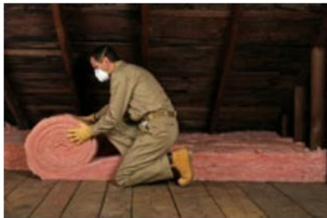
Air Seal & Insulate
