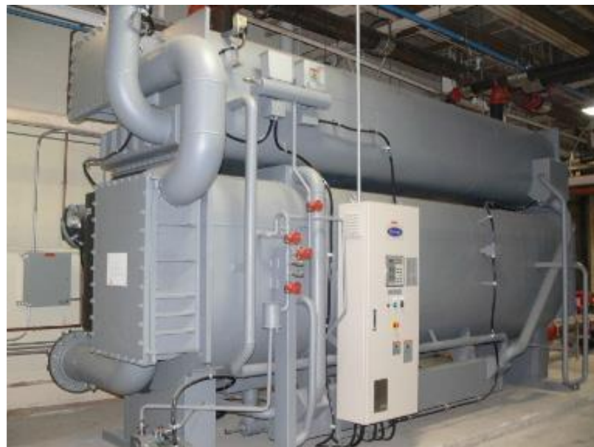
A 200-ton single-stage absorption chiller integrated with three 600 kW reciprocating engines that also provide hot water for process and space heating. The system is located at a metal fabrication facility in Fitchburg, Massachusetts. Photo courtesy of Northeast CHP Technical Assistance Partnership (CHP TAP).
